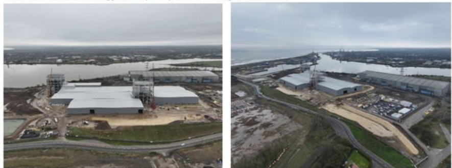
Northumberland Energy Park (NEP) 1 Site - Progress to date:
